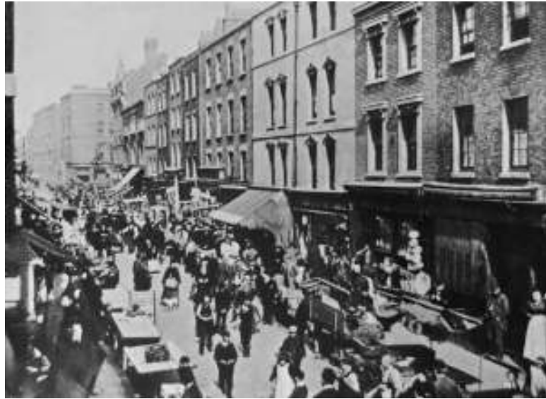
Looking up Brick Lane to Bethnal Green Rd - c.1900
