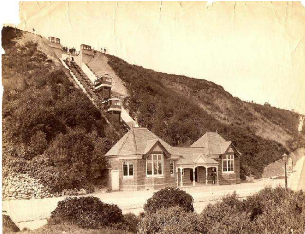
The lift originally employed a twin set of rails running for 50 meters, and had a gradient of 1:1.64.
